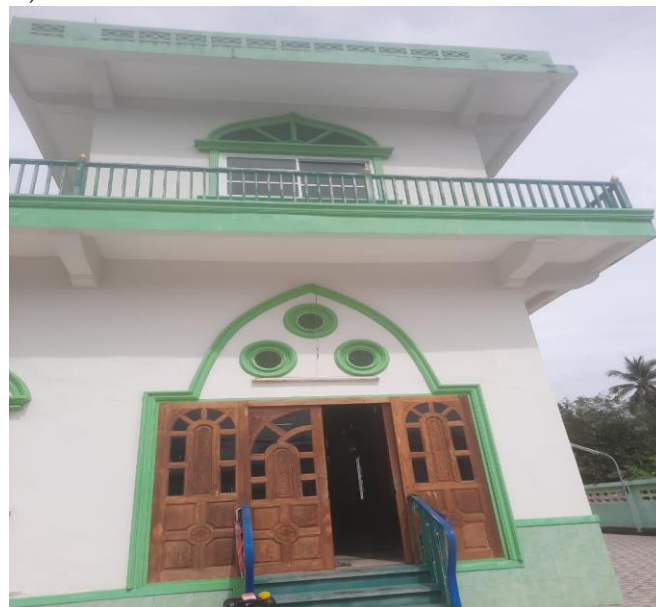
Figure 2. Condition of Darul Huda Mosque, field documentation, 2025.
