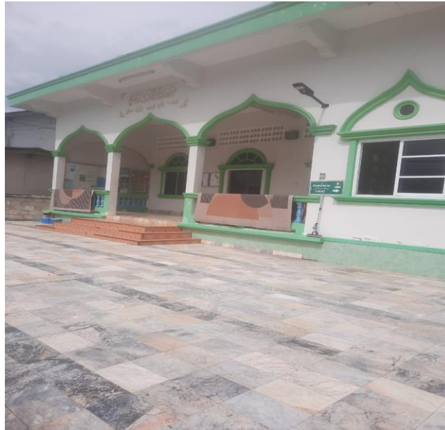
Figure 1. Condition of Darul Huda Mosque, field documentation, 2025.
